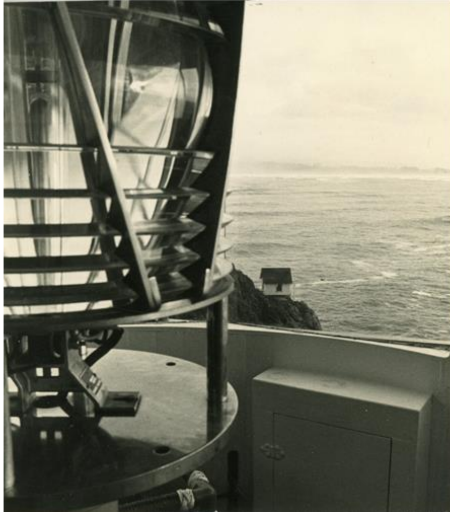
The 1947 Fifth Order Fresnel electric lens in the Trinidad Head Lighthouse with the 1898 Fog Bell House in the distance.
